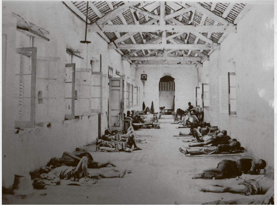
In 1894, Kennedy Town glassworks converted for use as a temporary hospital during the period of Hong Kong plague
