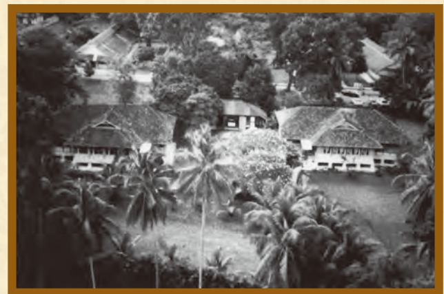
Fig. 10. TTSH Doctors' Residence at Akyab Road with teaching wards behind.
